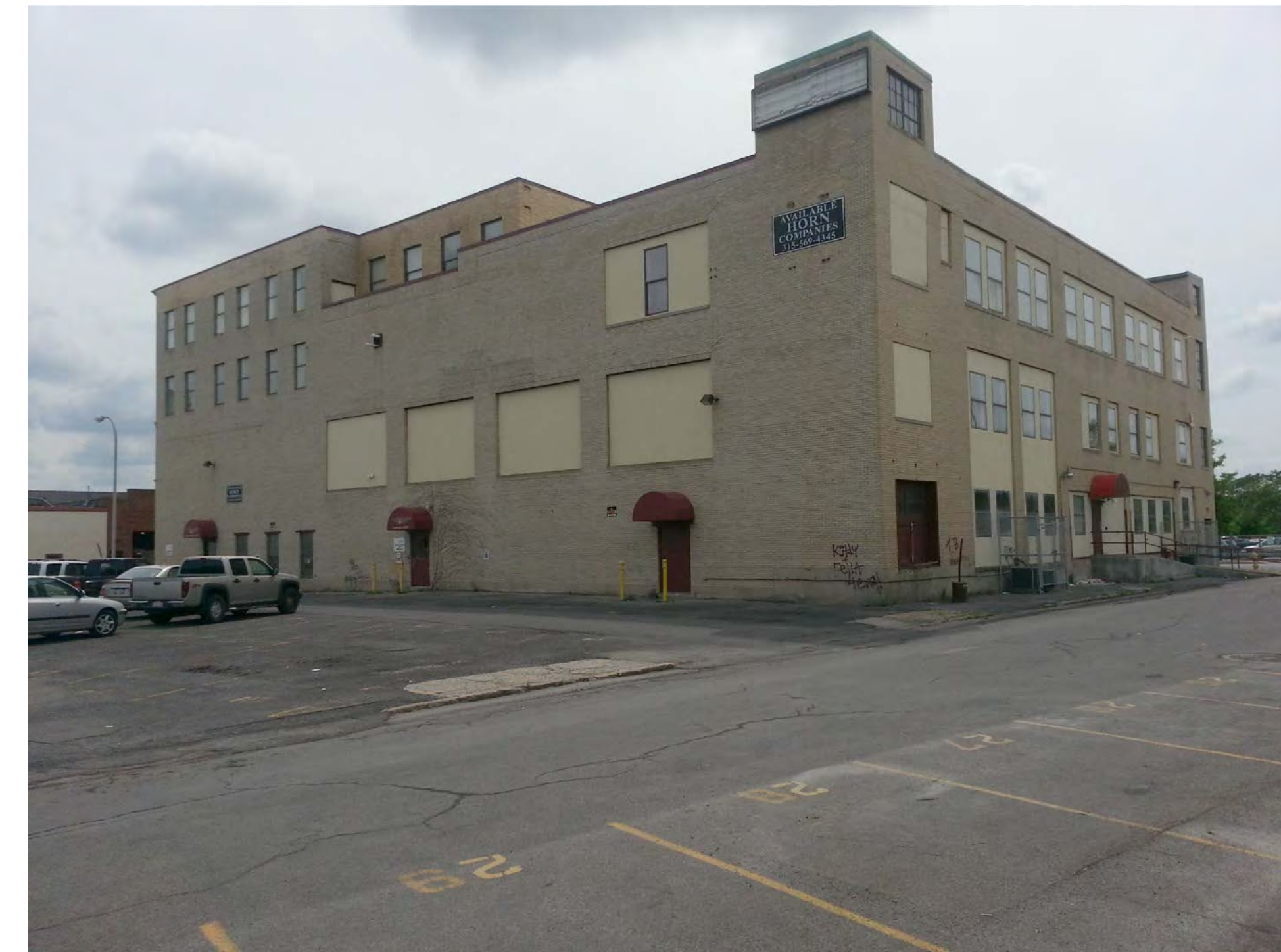
14 PHOTO LOOKING SOUTHWEST N.T.S.
